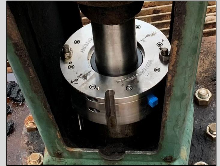
**After:** Split Air Mizer shaft seal installed using existing packing follower bolts
